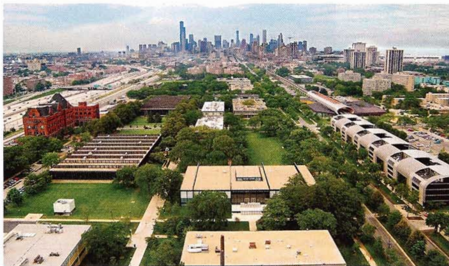
The Illinois Institute of Technology, shown here in an aerial view, is paying $12 million for its Perfect Power smart-grid electrical system. Photo courtesy of IIT
