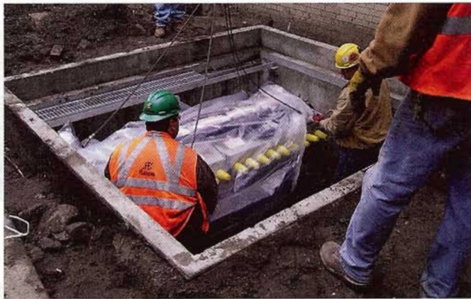
LEFT PHOTO: The Perfect Power system, illustrated by Michael Meiners with the Galvin Electricity Initiative, is a smart microgrid that serves a local area through dual electrical loops. RIGHT PHOTO: The advanced switchgear receives continuous feedback about the loop's condition and passes it to the master controller. Photo courtesy of IIT
